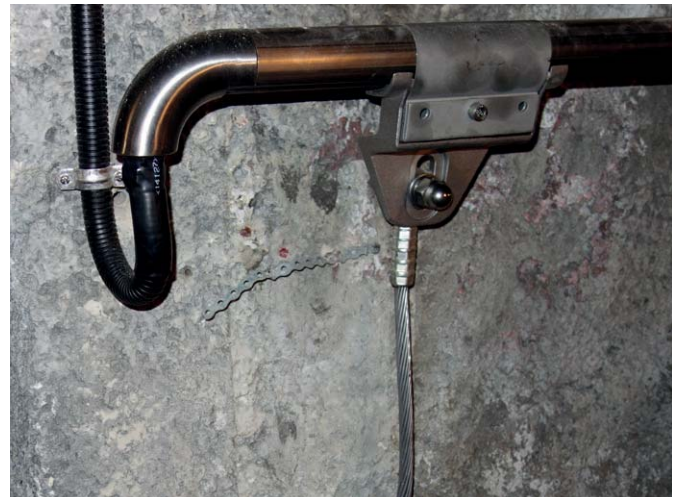
Curved end with cable gland
