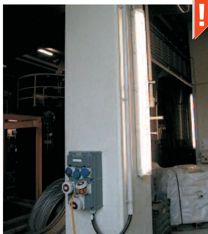
Vertical wall mounting with lampholder supports
