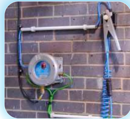
Earth-Rite® RTR road tanker truck static grounding system
