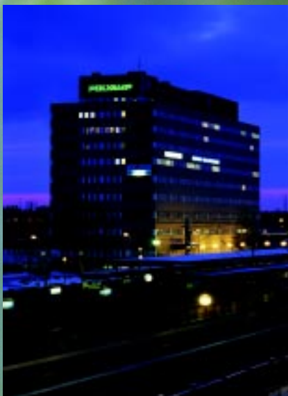
Head office and Systems Division in Sollentuna (Stockholm)
