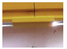
To do so, apply the protective bracket with the grip tab against the tunnel wall and push up until it latches noticeably.
