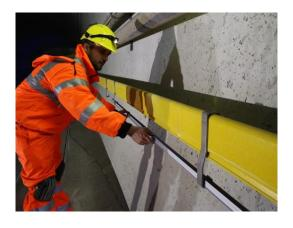
• Insert flat cable into the LaneLED unit from the bottom.
