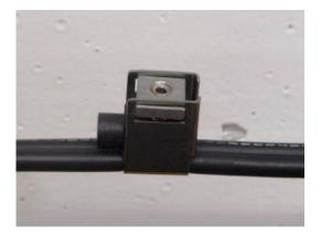
• Connect the LaneLED connection cable to the current collector with the white markings at the top.
