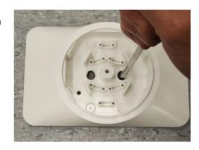
Hold the surface-mounted adapter in the required mounting position on the shoulder and mark the drill holes with a marker pen or a 5mm concrete drill bit.
