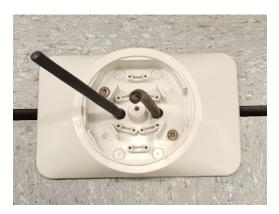
Strip back the connection cables ~12cm and remove insulation ~11mm.
