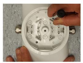
Apply a closed circular bead of Permafix adhesive to the rear of the surface-mounted adapter.
