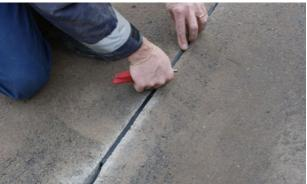
The area of the MarkLED must be cast with liquid hot bitumen.
