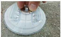
Screw MarkLED with countersunk screw 4.5x50 item no. 17473 onto the ground.
