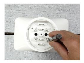
Apply a circular bead of Permafix adhesive to the bottom of the surface-mounted adapter with an open section facing the tunnel wall.
