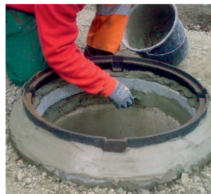
Time-saving Installation of a manhole cover with PCI Polyfix plus.
